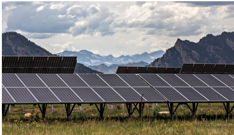
Solar panels at the National Renewable Energy Laboratory in Golden, Colorado. Credit: Werner Slocum / NREL
